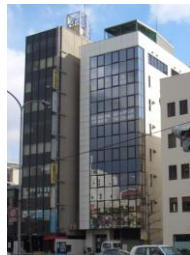
Daikai Bldg. annex
