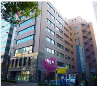
Takamatsu Bancho Bldg.
